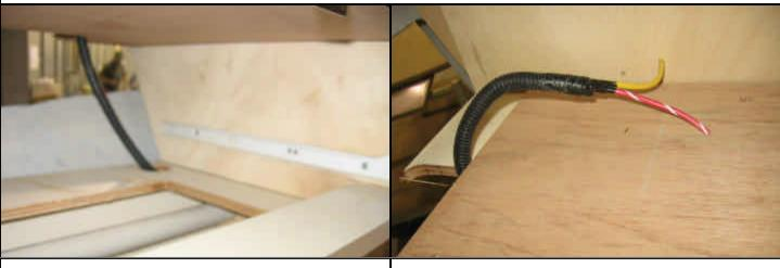
Fig.4 Pull the freezer wires from sub floor cutout, run the wires upward. Fig.5 Run the wires to freezer compartment, for further installation.
